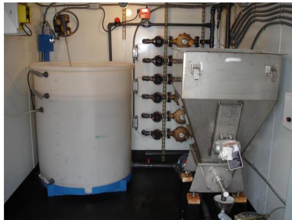
The ISD™ system was fabricated and installed by ETEC, and was able to re-circulate over 2.3 million gallons of groundwater over a 3 month timeframe (~35 gpm rate) and amend it with 8,200 lbs of CarBstrate™. Groundwater was extracted from 11 extraction wells (blue EWs), automatically amended with CarBstrate™, and distributed into the subsurface via 20 injection wells (orange IWs).
